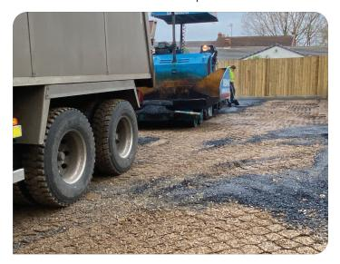
CORE TRP provided a robust solution by creating a load-bearing, porous subbase that protected tree roots while satisfying all regulatory standards. The system's 200mm depth ensured the road could support heavy vehicles, making it suitable for adoption by the local authority.
