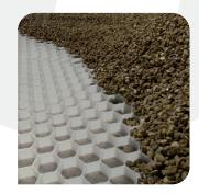
Install the grid starting from one corner and working your way out with the membrane facing down. Cut to shape using a petrol disc cutter or grinder. Please ensure to wear necessary PPE for the equipment being used. Fill the grid with your chosen aggregate either using a wheelbarrow or direct from a truck.
