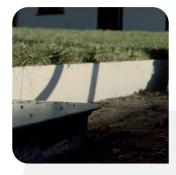
Install a suitable edging around all open sides. This could be tanalised wood edging, block paviours, granite setts or our very own edging variations (CORE PRO EDGE shown here). Ensure to set your edging height 15-20mm higher than the grid level to prevent the dressing layer spilling out onto surrounding areas.
